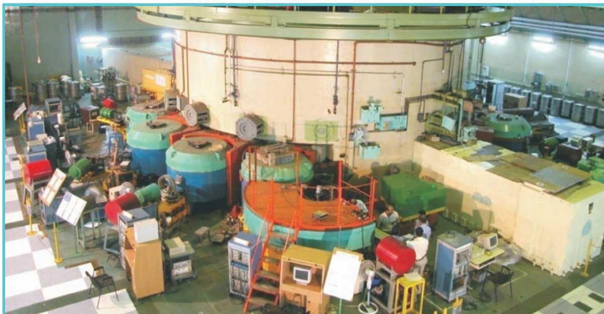
Fig. 3. A view of neutron scattering facilities inside the Dhruva reactor hall
